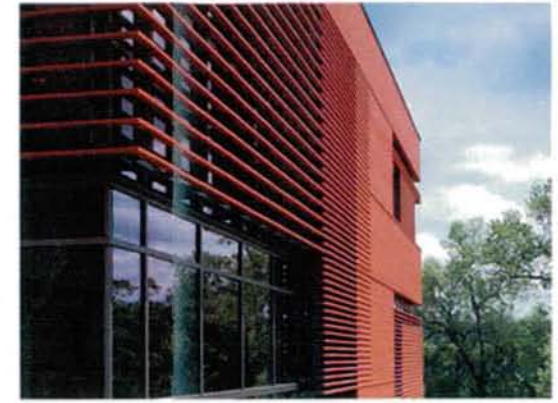
Sunshading and Curtainwall
