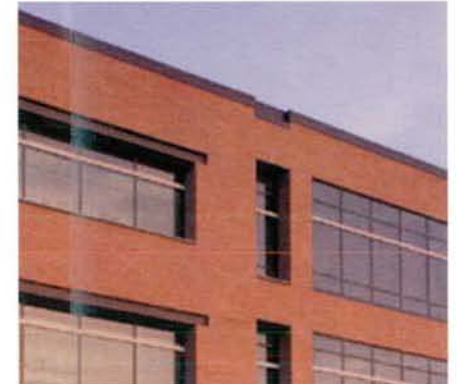
Brick Masonry with Punched Windows
