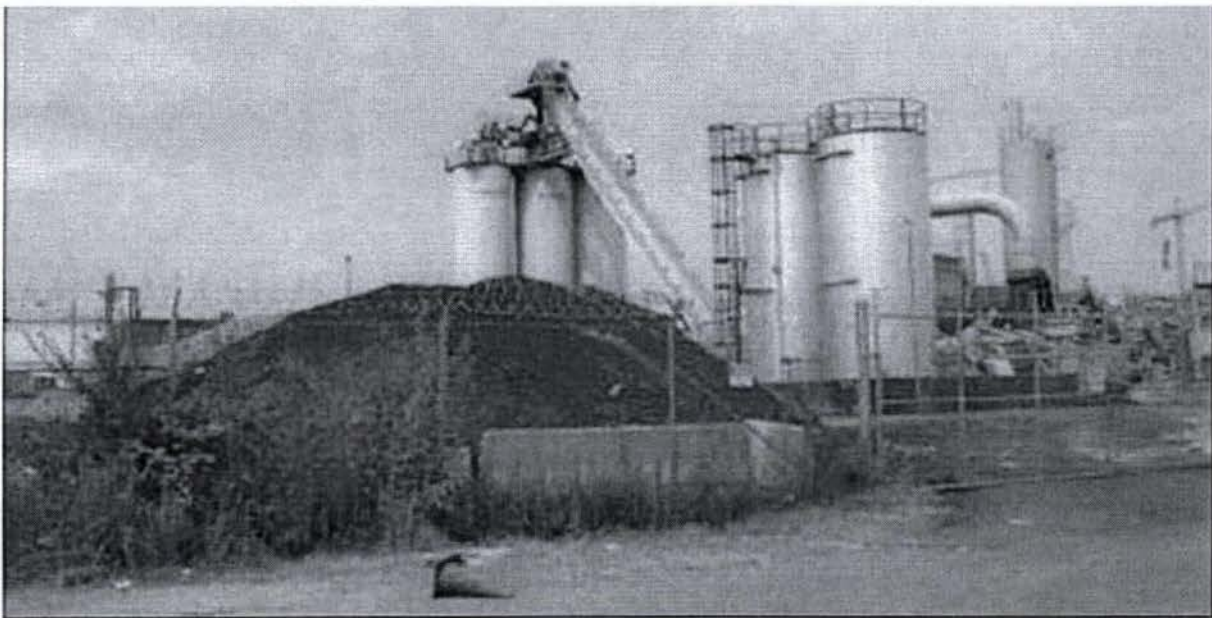
Context: Asphalt Manufacturing Process at Existing Plant
