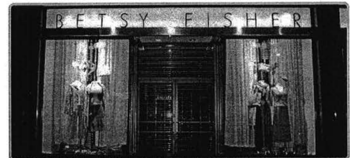
BETSY FISHER - (DUPONT CIRCLE) NOTE USE OF THE INTERIOR WIRE MESH SECURITY GRILL
