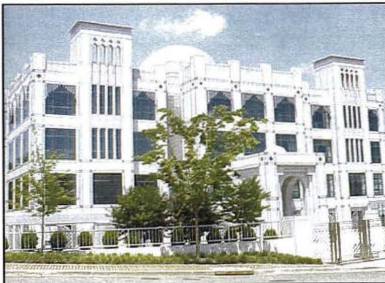
Chancery of the United Arab Emirates in the International Chancery Center
