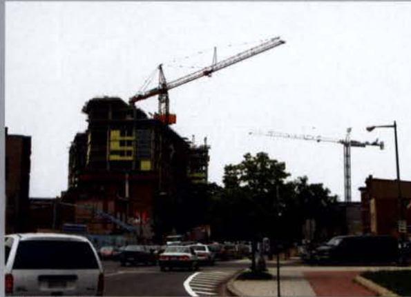
Additional residential construction on Massachusetts Avenue
