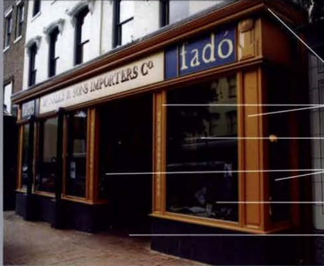
5th Street Ground Floor Facades
