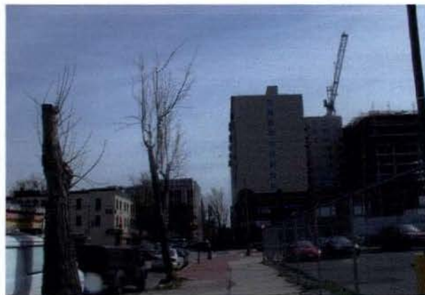
Illustration 2: Looking South on 5 th Street from L Street toward K Street.. Square 483 is in foreground on the right. Square 484, with the Monarch Paint Building is on right, mid-ground
