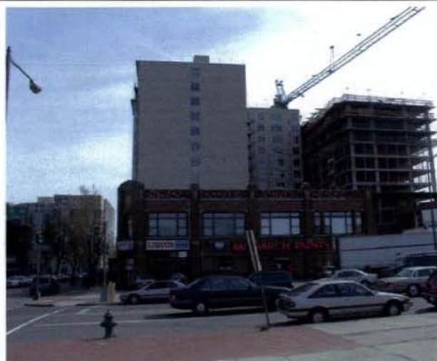
Illustration 4: Looking South from Square 483 to Square 484. Monarch Paint Building is low building in mid-ground.
