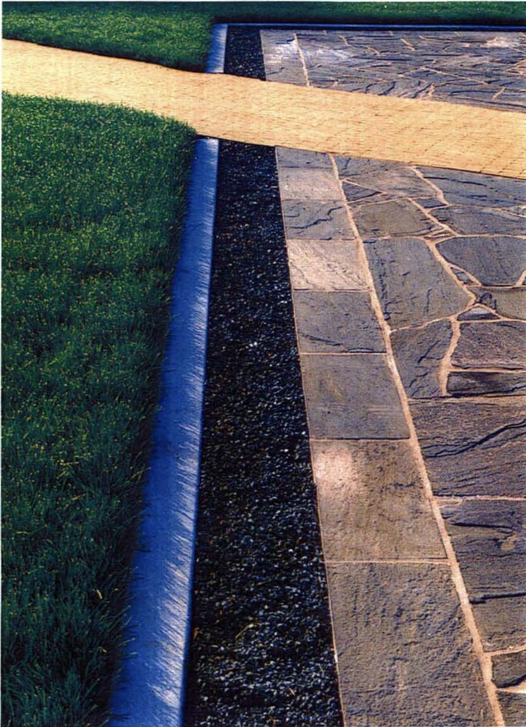
A stone edge collects and conveys runoff from the adjacent paved area to be conveyed to a bio-filtration bed.
