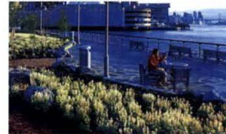
4. PAVEMENT GRADED TOWARD BIO-FILTRATION BEDS
