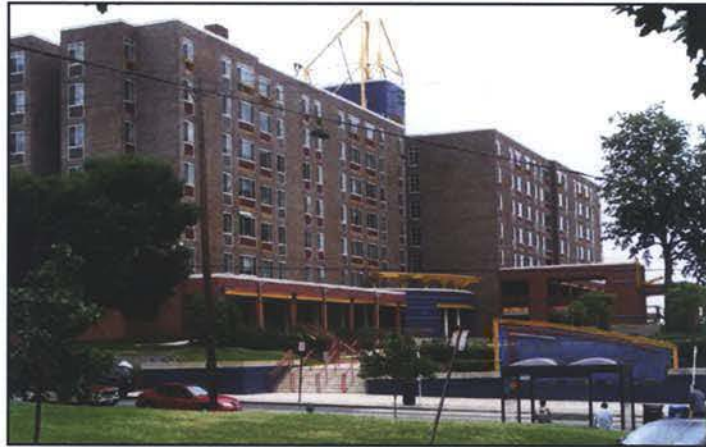
Edgewood Terrace – 601 Edgewood Terrace
