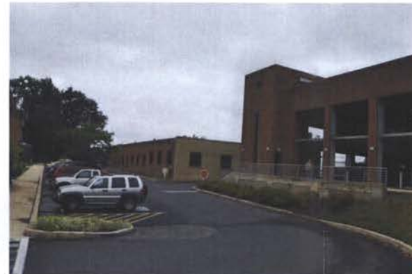
DRIVE AND PARKING GARAGE WEST OF DENISON HOUSE
