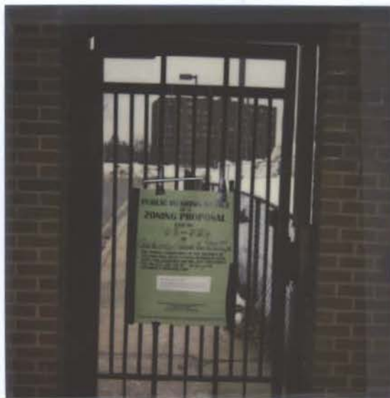
2-15-10 Replacement West Virginia Ave East Gate
