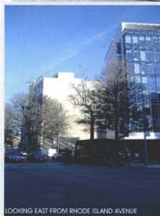
LOOKING EAST FROM RHODE ISLAND AVENUE
