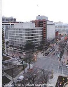
LOOKING WEST AT RHODE ISLAND AVENUE
