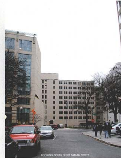
LOOKING SOUTH FROM BASAN STREET
