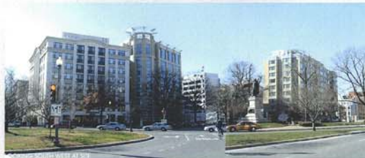
LOOKING SOUTH FROM SITE
