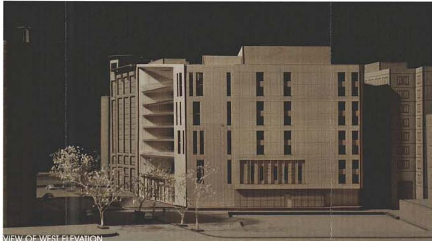
VIEW OF WEST ELEVATION
