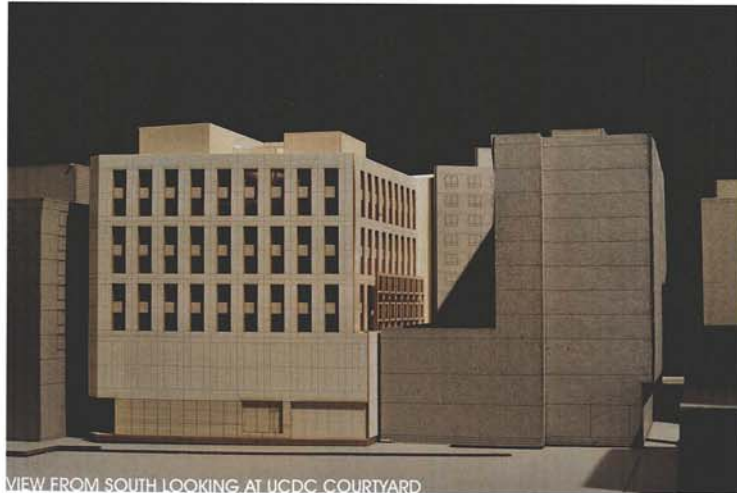
VIEW FROM SOUTH LOOKING AT UCDG COURTYARD
