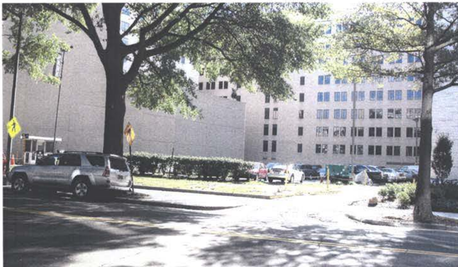
Subject's Parking Lot and Alley at Western Elevation
