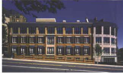
Extended Wall at Screen And Chimney Enclosures at Vents
