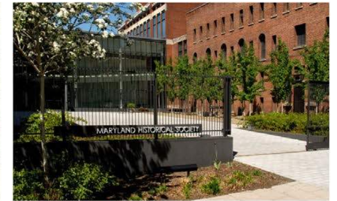
DECORATIVE FENCE AND SLIDING GATES
