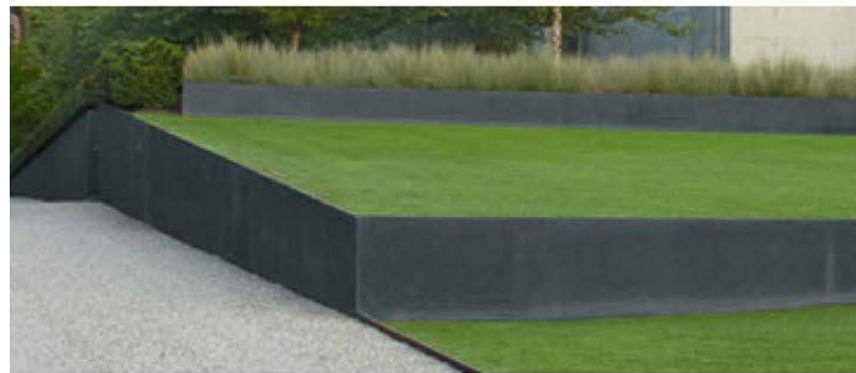
STEEL RETAINING WALLS
