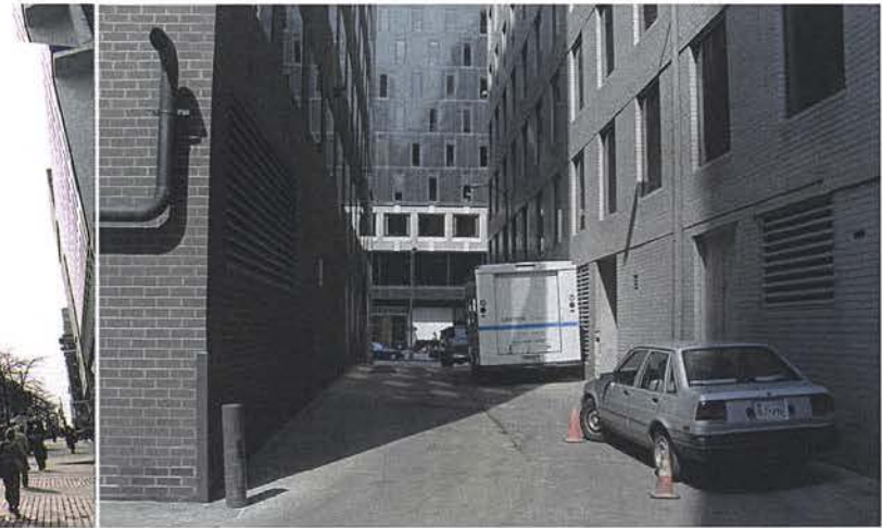
6: View of 20' Alley at Square 126 Looking West to 18th Street
