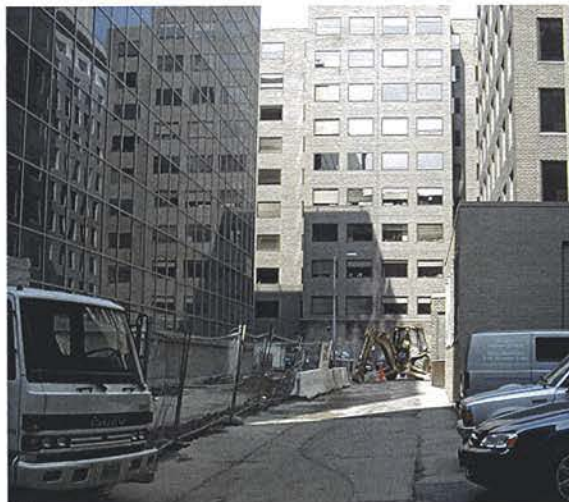
10: View of 20' Alley at Square 126 Looking West from Barr Building
