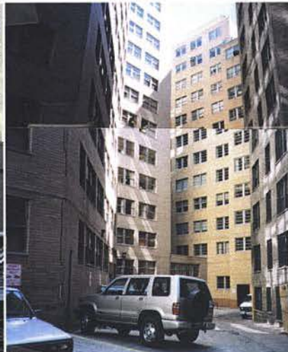
11: View Towards Alley Cul-de-sac Between Lot 56, 851 and Barr Building From 20' Alley at Square 126
