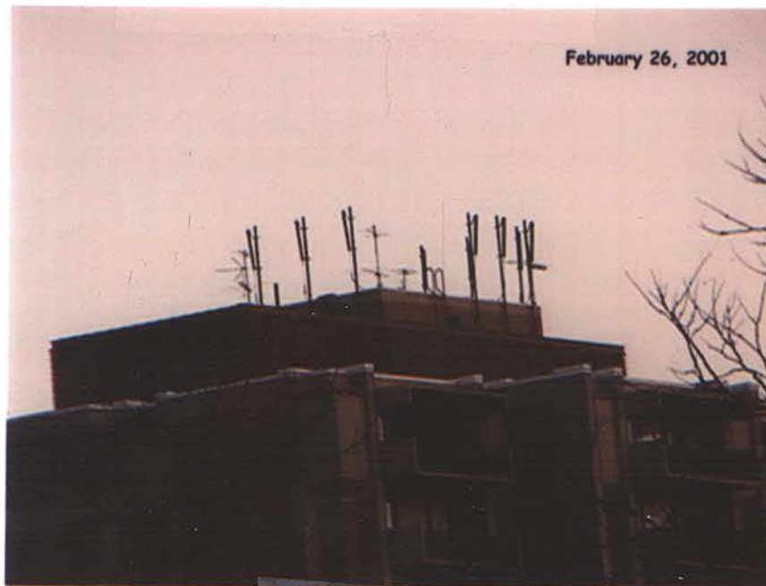
Rooftop of 2440 Virginia Avenue, NW
