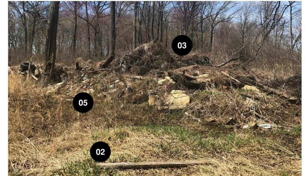
EXISTING SITE PHOTO-03
