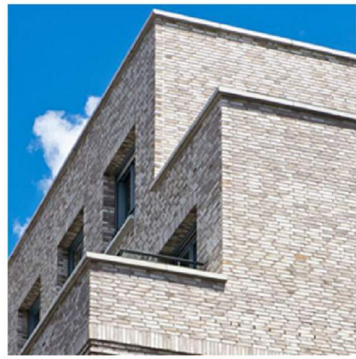
A BRICK MASONRY
