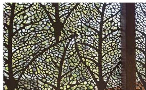
5. LASER-CUT MTL PANEL
