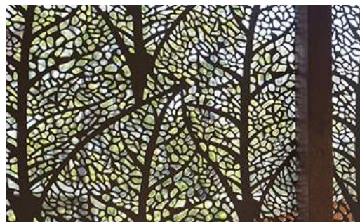
5. LASER-CUT MTL PANEL RAILING SYSTEM
