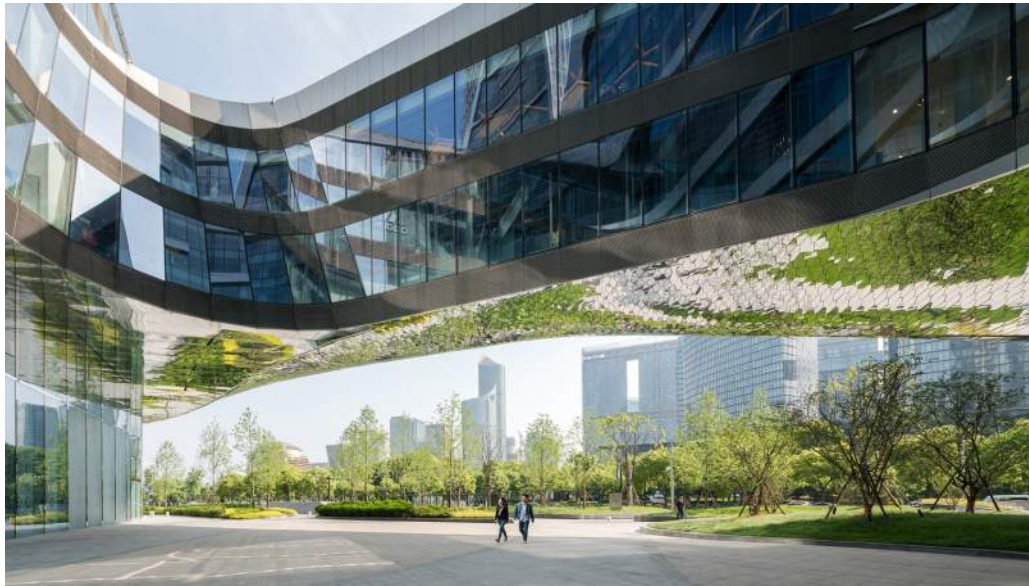
7. REFLECTIVE ALUMINUM CLADDING PANELS
