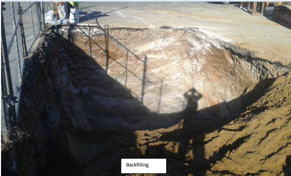
4 ft wide western extension of excavation
