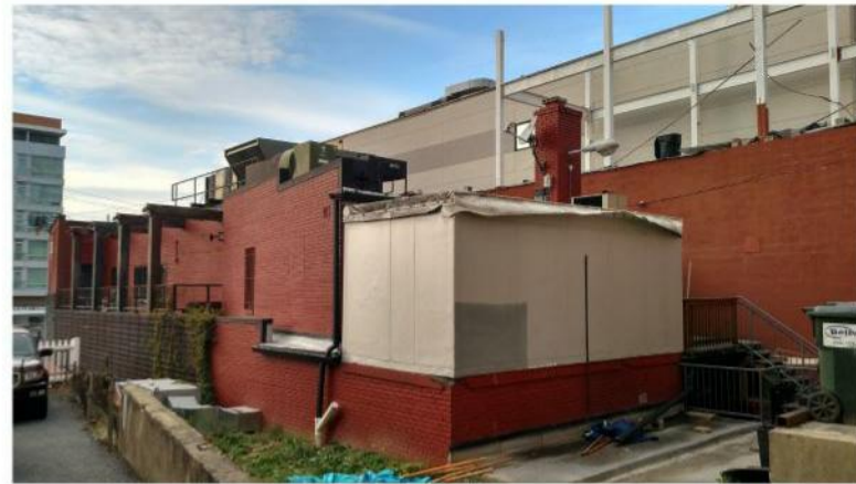
4. View from alley looking northwest
