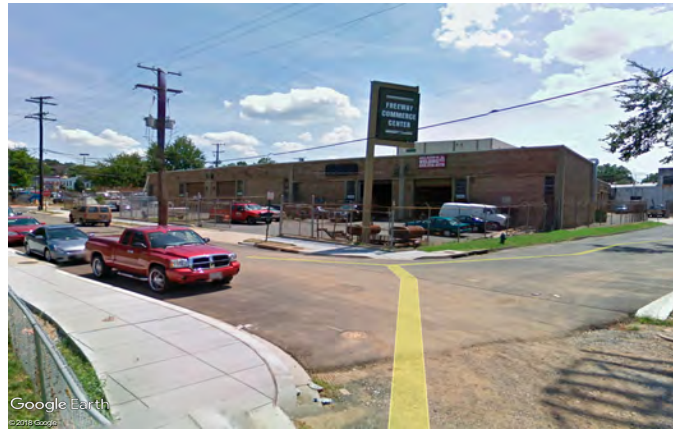
① LOOKING SOUTH FROM RAILROAD AVE AND W ST.
