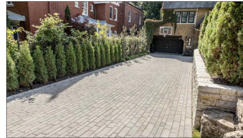
TYPICAL PERMEABLE CONCRETE PAVER FOR RESIDENCE DRIVEWAYS
