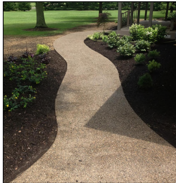
CONCRETE WITH AGGREGATE WALKWAYS
