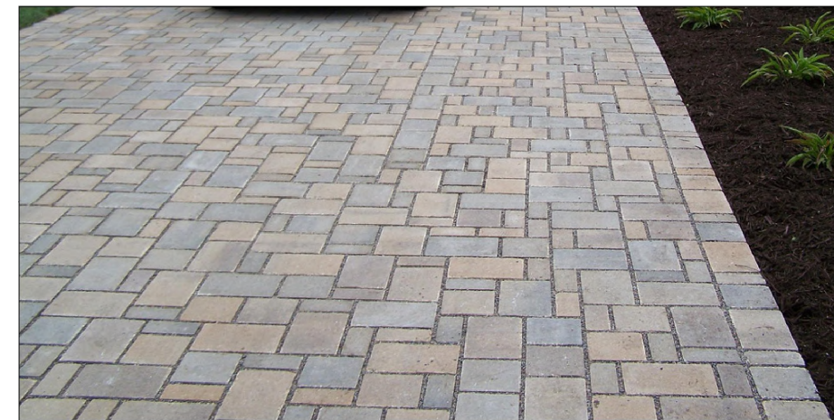
TYPICAL PERMEABLE CONCRETE PAVER FOR MAIN DRIVEWAY
