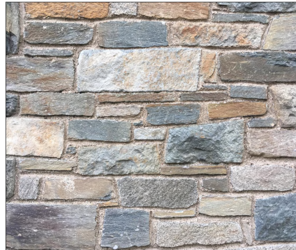
FIELDSTONE FACADE ON EXISTING HOME TO MATCH FOR RESIDENCES AND SITE WALLS
