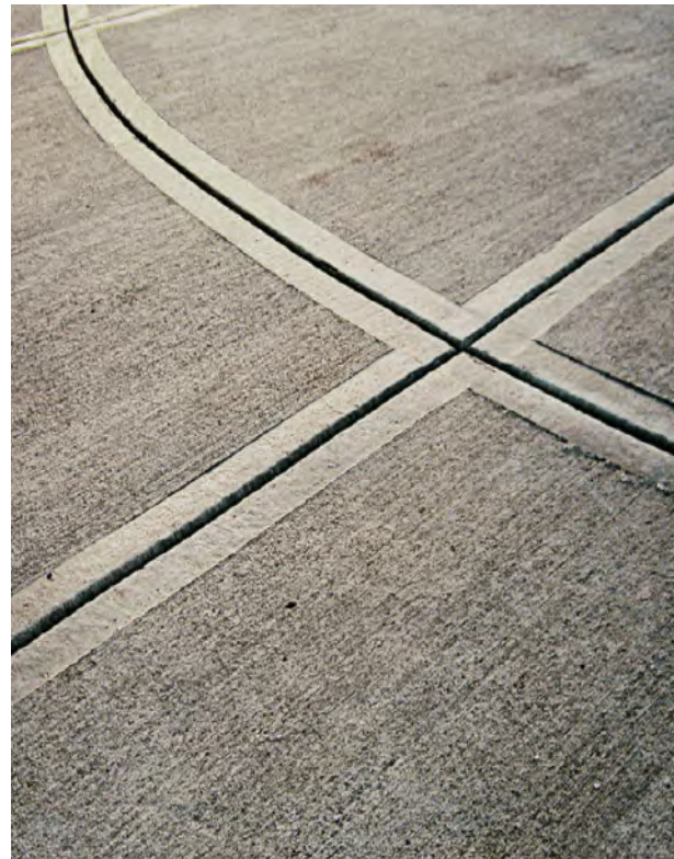
CONCRETE SIDEWALK: 3'x3' Scoring, Hairbroom Finish
