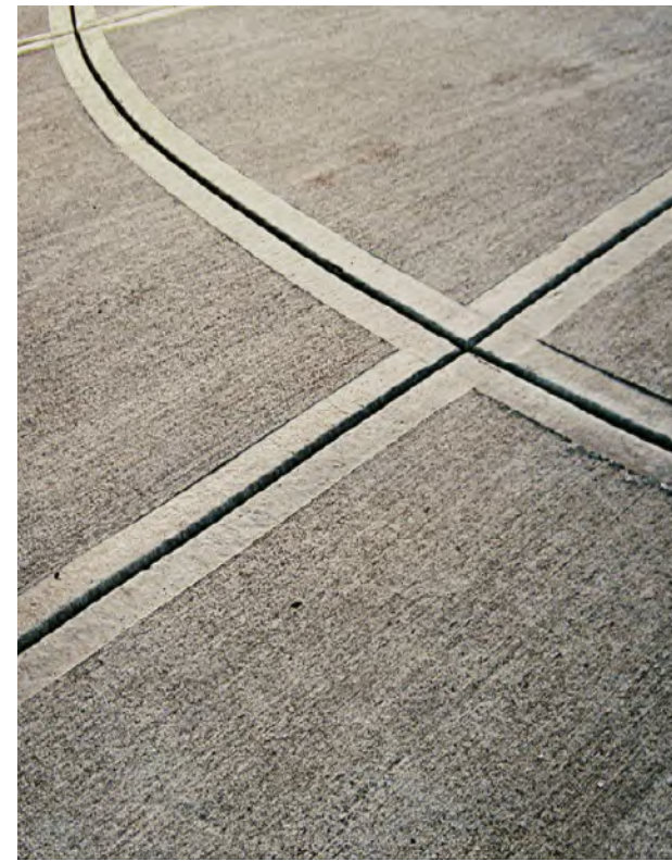
CONCRETE SIDEWALK: 3'x3' Scoring, Hairbrush Finish
