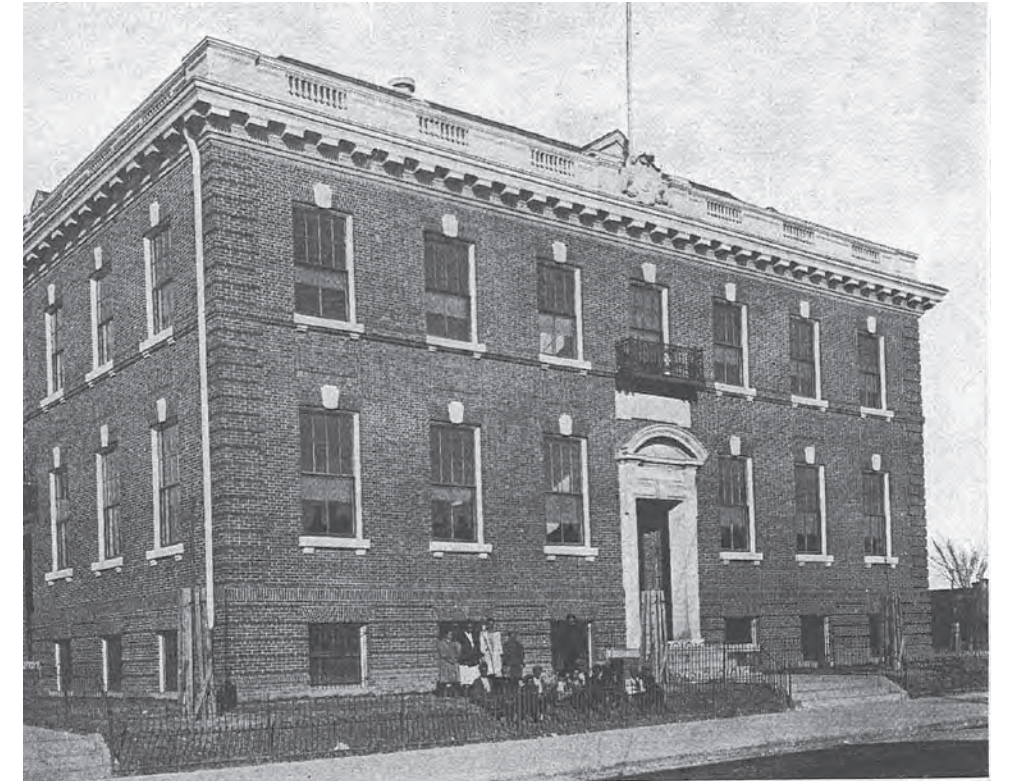
CENTRAL BUILDING PHOTOGRAPH (1908)- ROLLED CURB
