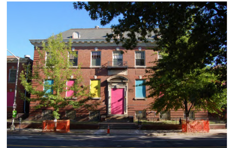
SOUTH ELEVATION (EXISTING CONDITIONS)
