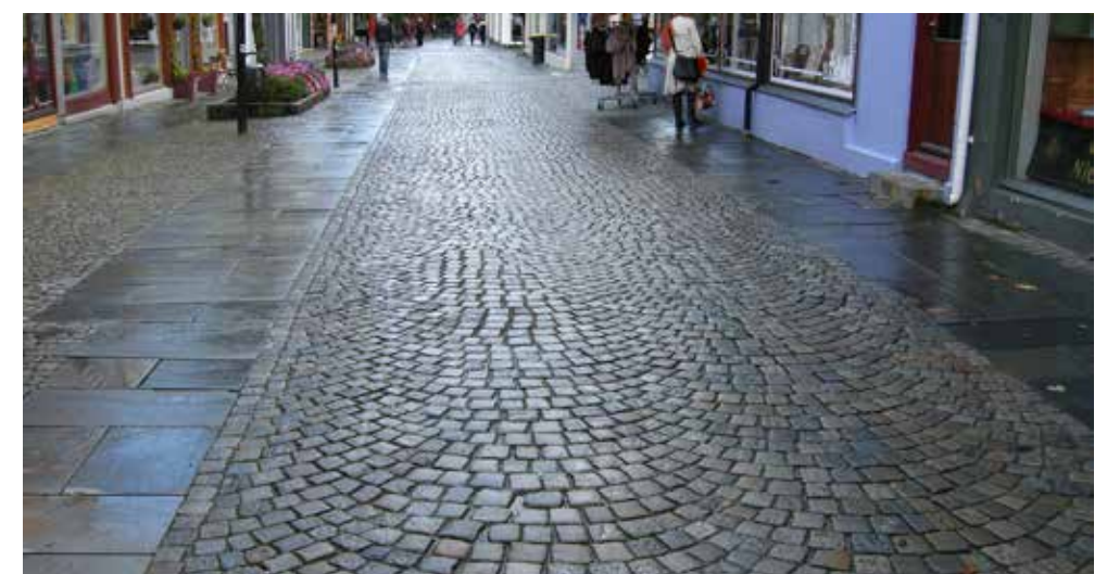
Curbless Paving and Vehicular Overlapping Paving
