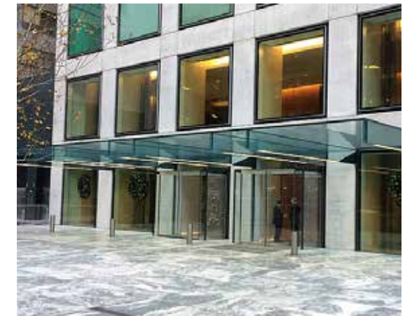
5. DROP-OFF CANOPY CLEAR STRUCTURAL GLASS
