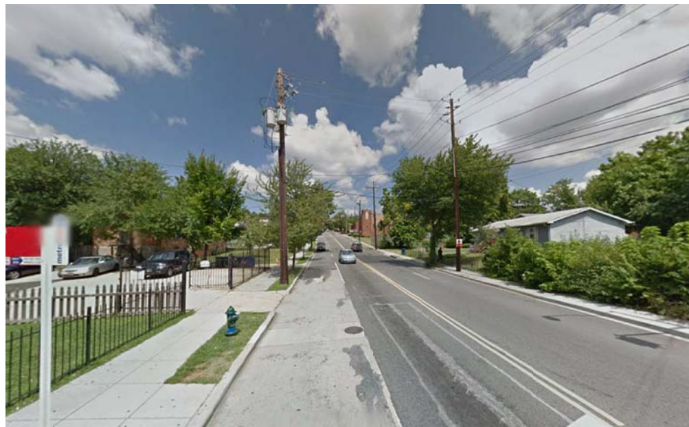
3 - VIEW NORTH DOWN DIVISION AVE NE
