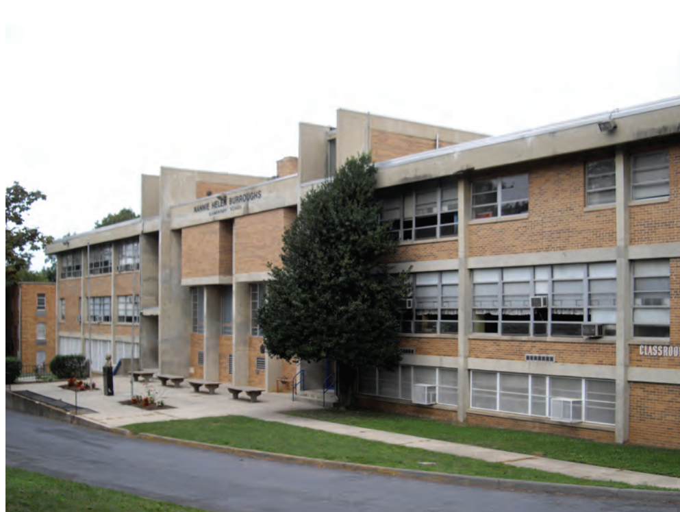
H School Building
