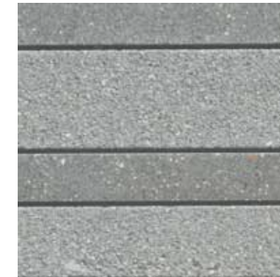
Ground-Face CMU Wall Linear Pattern
