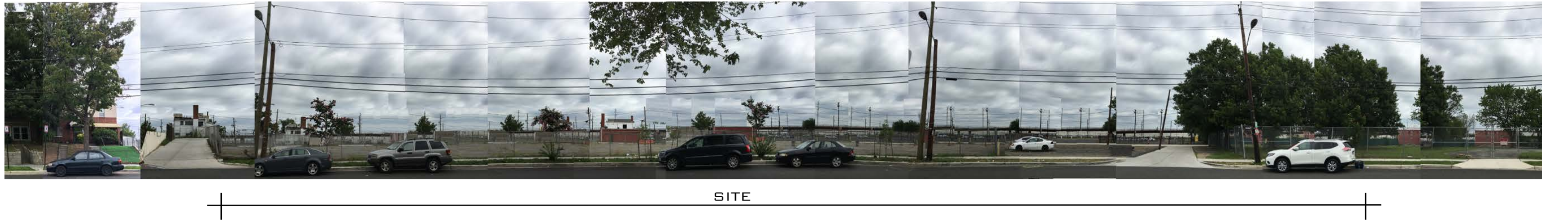
1 | EADS STREET ELEVATION LOOKING NORTH
