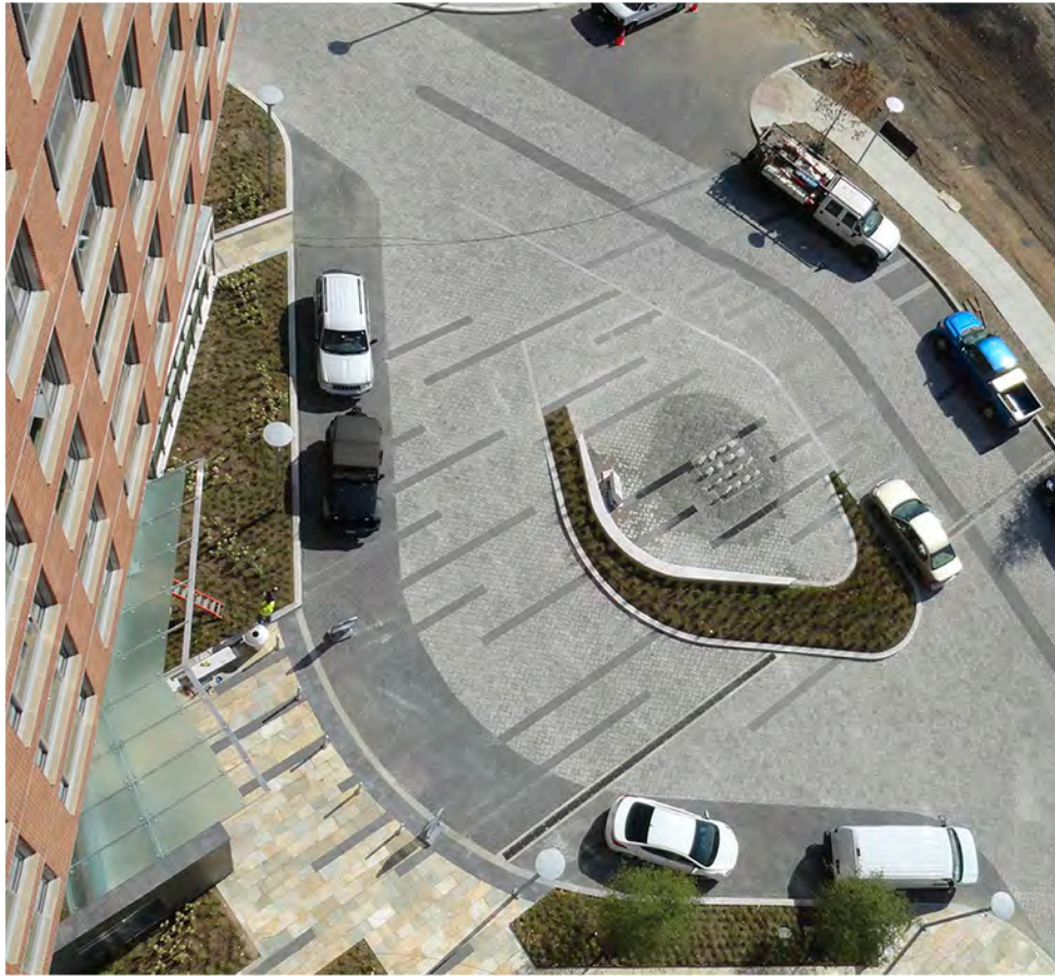
Plaza and sidewalk paving
