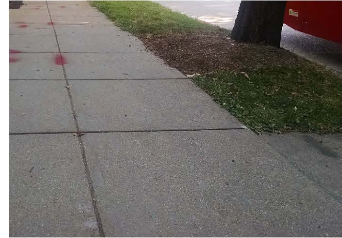
DC STANDARD CONCRETE PAVING
