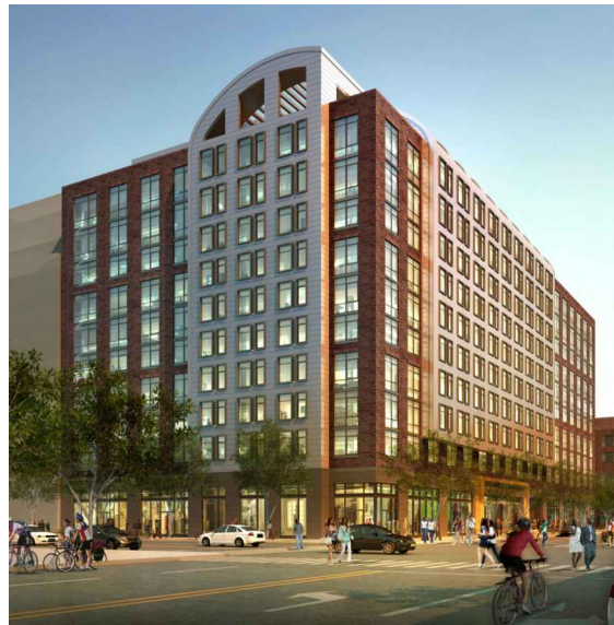
500 & 530 morse st. NE -9 story / 270 du's -20,000 Sf. Retail Pending Development
