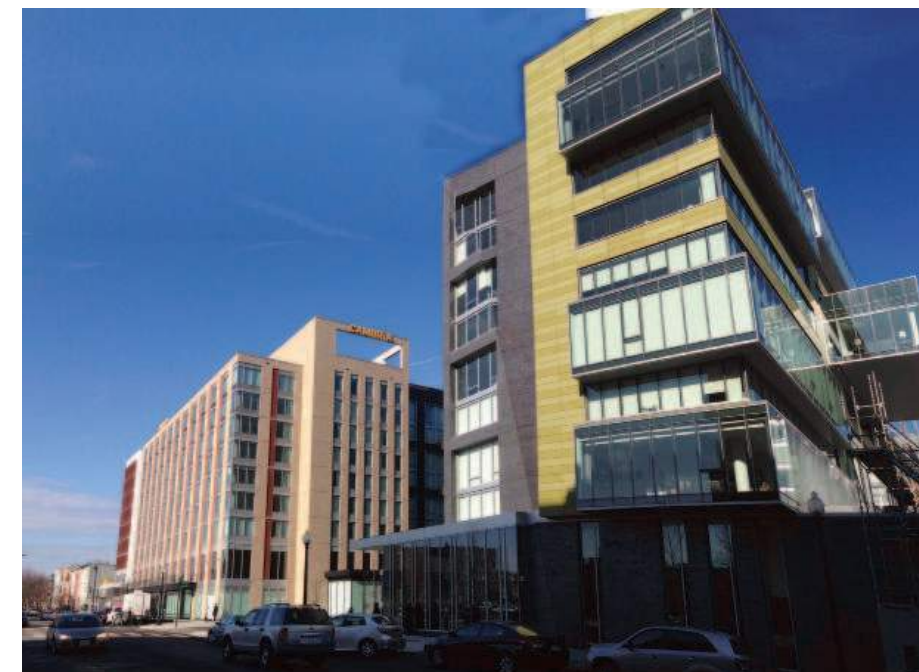
7 O Street NW - Looking NORTHWEST
