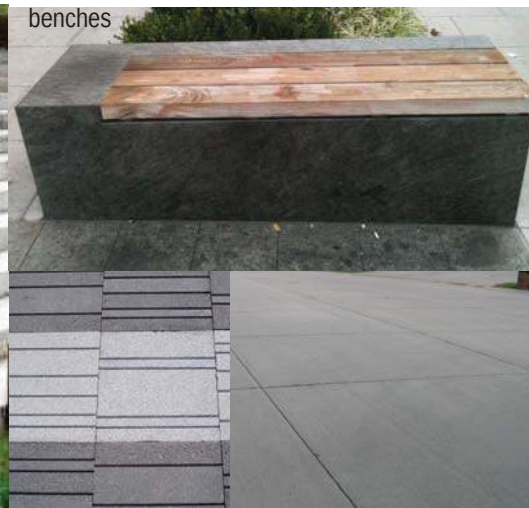
benches special paving scored concrete on ADA path
