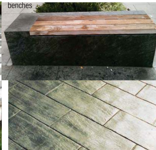
stamped concrete on ADA path
