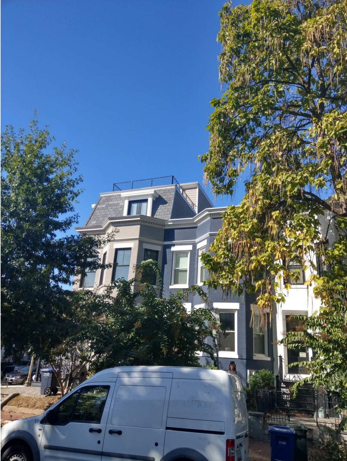
900 11 th Street NE – Third Floor Addition with Roof Deck and Penthouse Access Front Elevation (Taken from 11 th St NE)
