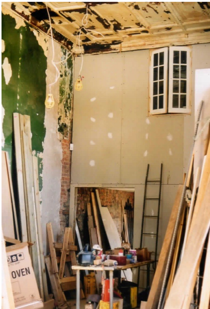
Mezz. (rebuilt) from Gallery - 2001
