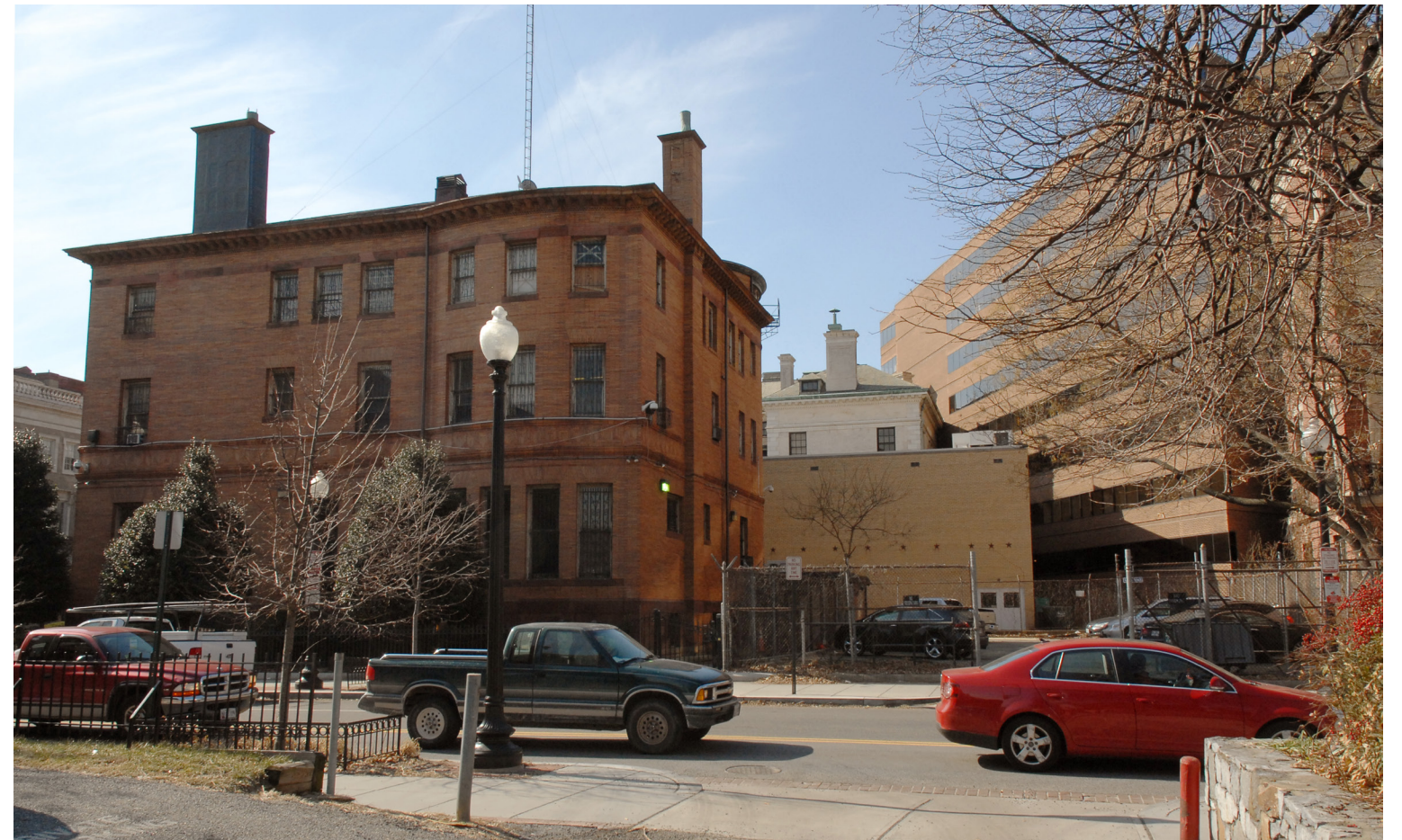
View from 18th Street
