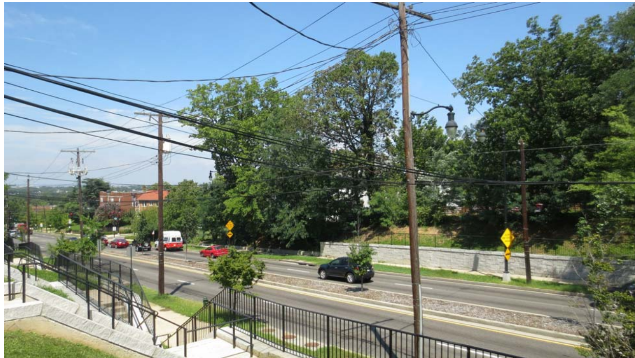
EXISTING SITE CONDITION - PENNSYLVANIA AVE., SE
