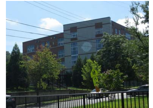
RANDLE HIGHLANDS ELEMENTARY SCHOOL - 1650 30TH ST, SE 4 STORIES
