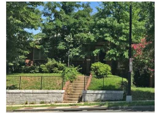
RESIDENCE - 2920 PENNSYLVANIA AVE, SE 1 STORY
