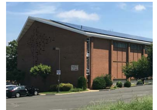
PENNSYLVANIA AVE BAPTIST CHURCH - 3000 PENNSYLVANIA AVE, SE 3 STORIES
