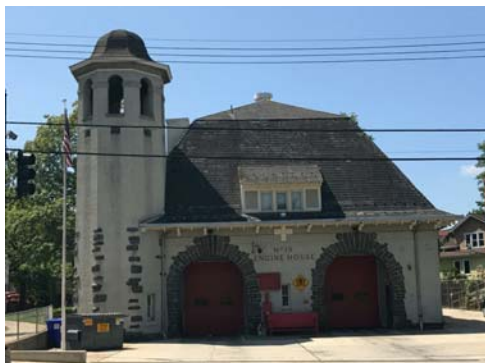
ENGINE CO. NO. 19 FIRE & EMS STATION - 2813 PENNSYLVANIA AVE, SE 2 STORIES
