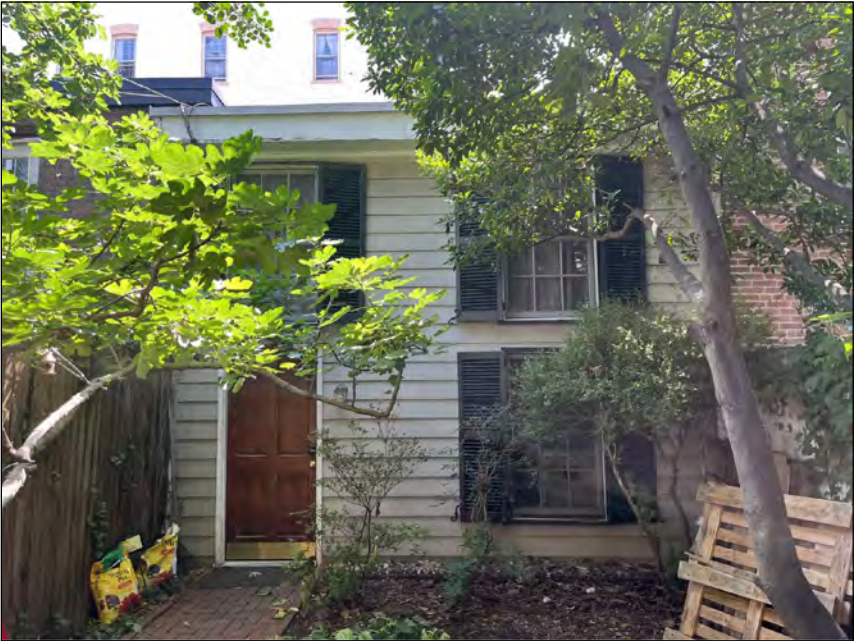
EXISTING REAR YARD VIEW
