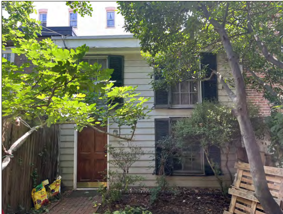
EXISTING REAR YARD VIEW LOOKING EAST
