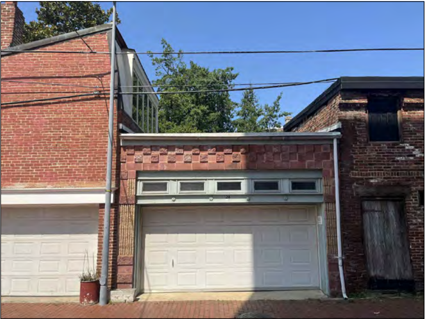
EXISTING ALLEY VIEW
