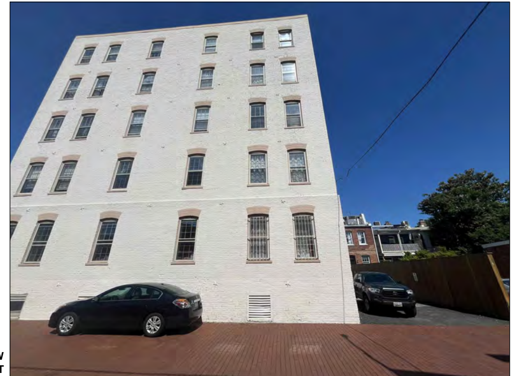
EXISTING ALLEY VIEW LOOKING EAST
