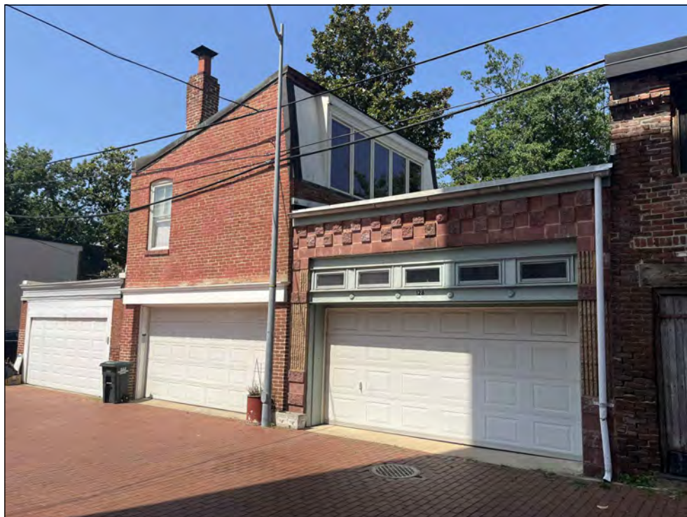
EXISTING ALLEY VIEW LOOKING SOUTH-WEST
