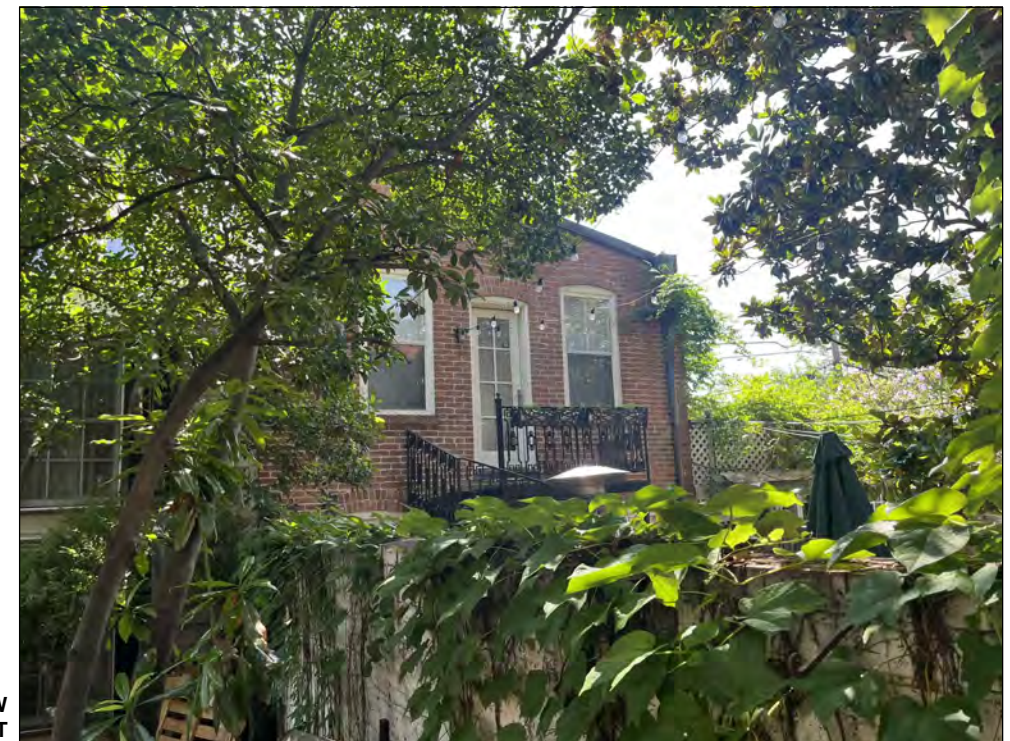
EXISTING REAR YARD VIEW LOOKING SOUTH-EAST
