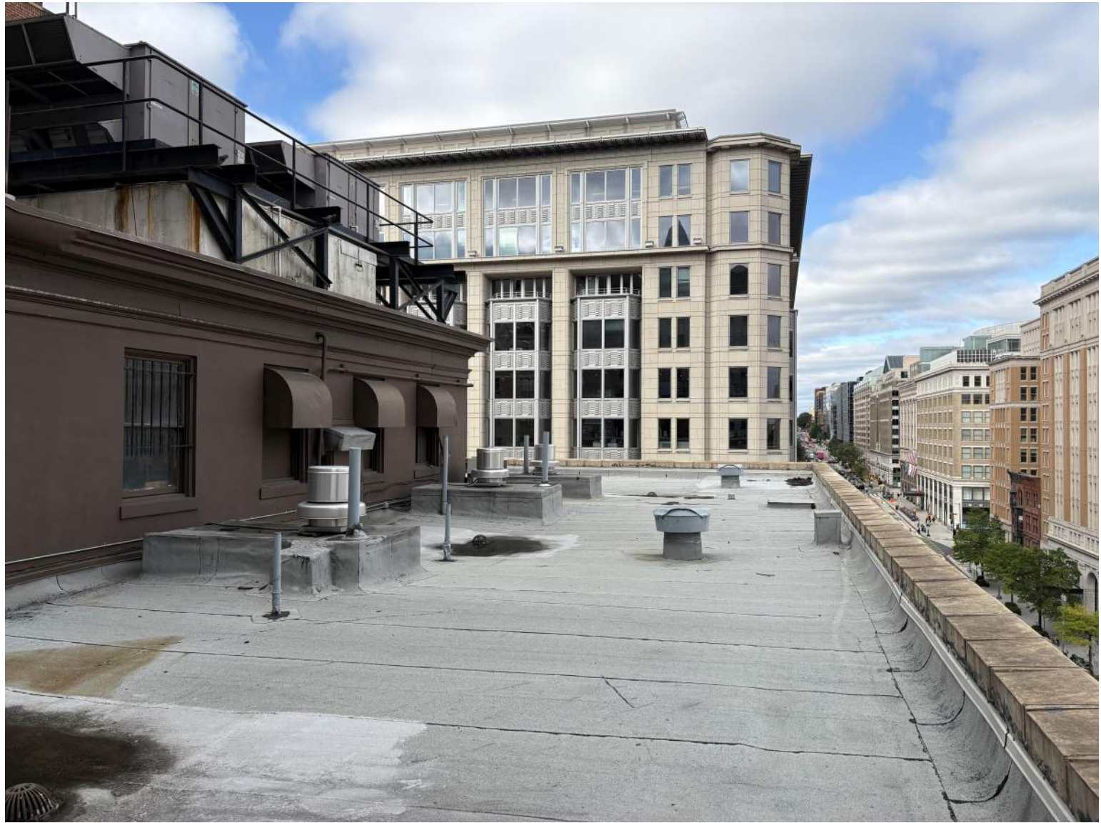
8TH FLOOR ROOF - LOOKING NORTH ON 11TH ST
