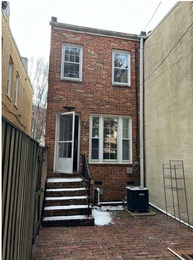
Exterior: Rear wall, windows, and door to be demoed
