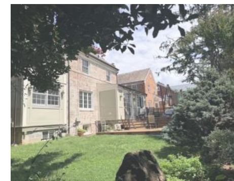
SOUTH WEST VIEW
