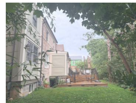
WEST VIEW (FROM 47TH ST/ OVER FENCE)
