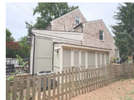
EAST VIEW (SOUTH END)
