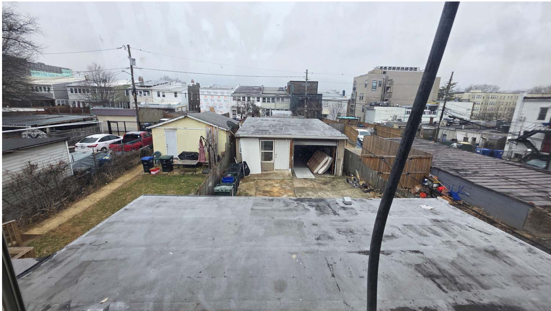
VIEW TOWARDS REAR ALLEY
