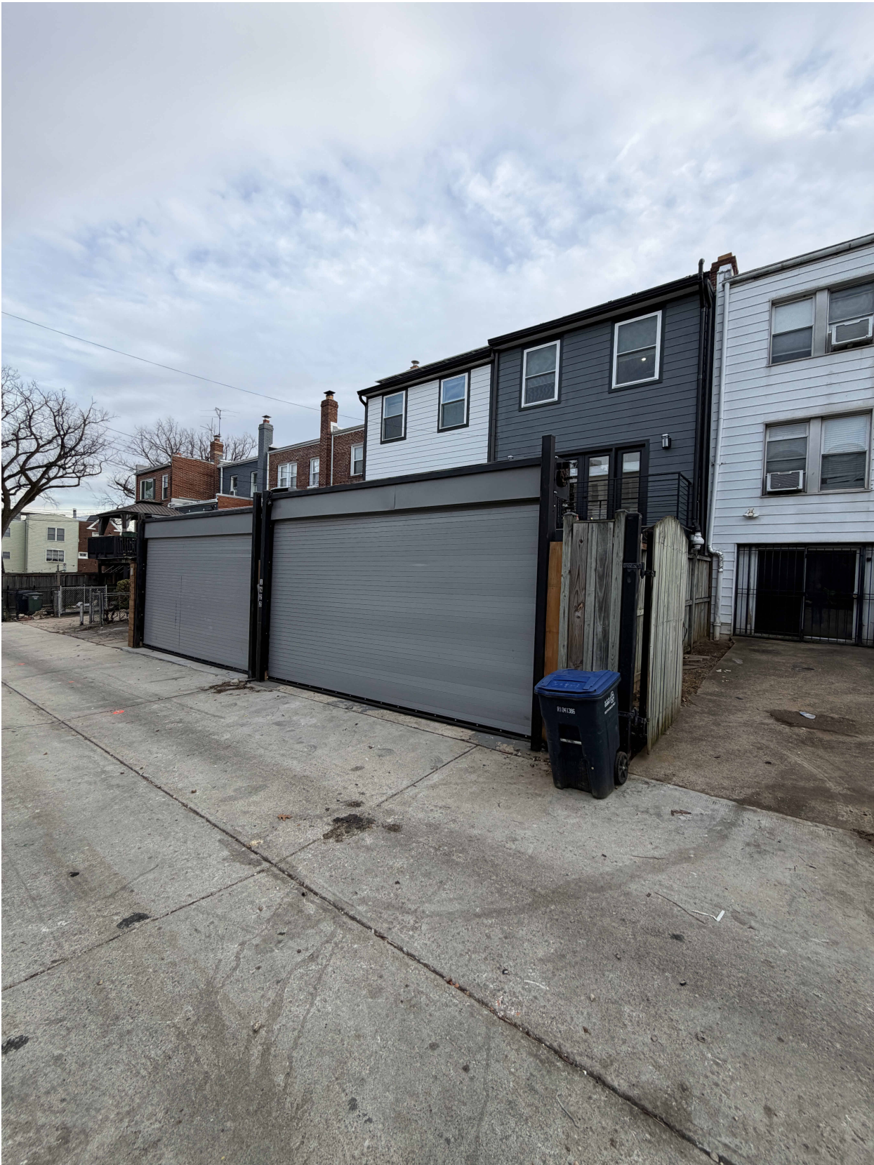
3 EXISTING CONDITIONS - VIEW LOOKING FROM ALLEY EAST NTS
