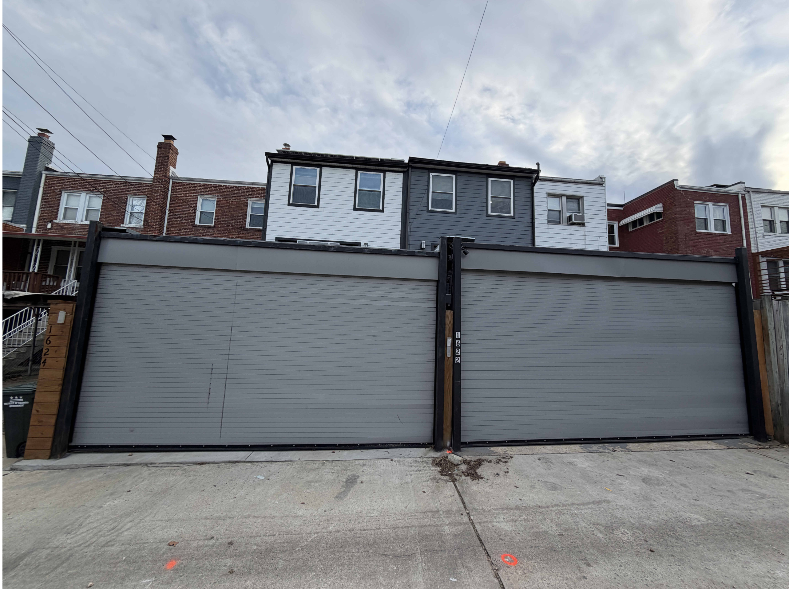
1 EXISTING CONDITIONS - VIEW LOOKING FROM ALLEY NTS
