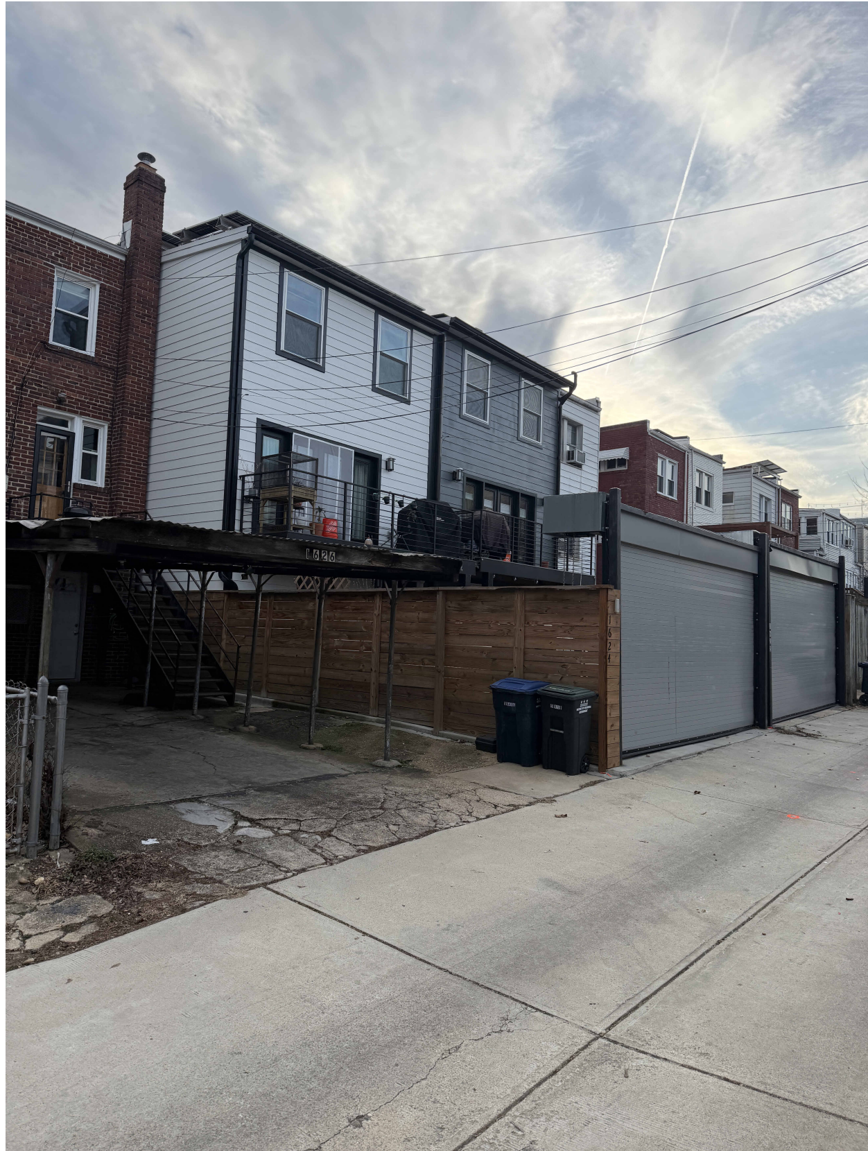
2 EXISTING CONDITIONS - VIEW LOOKING FROM ALLEY LOOKING WEST NTS
