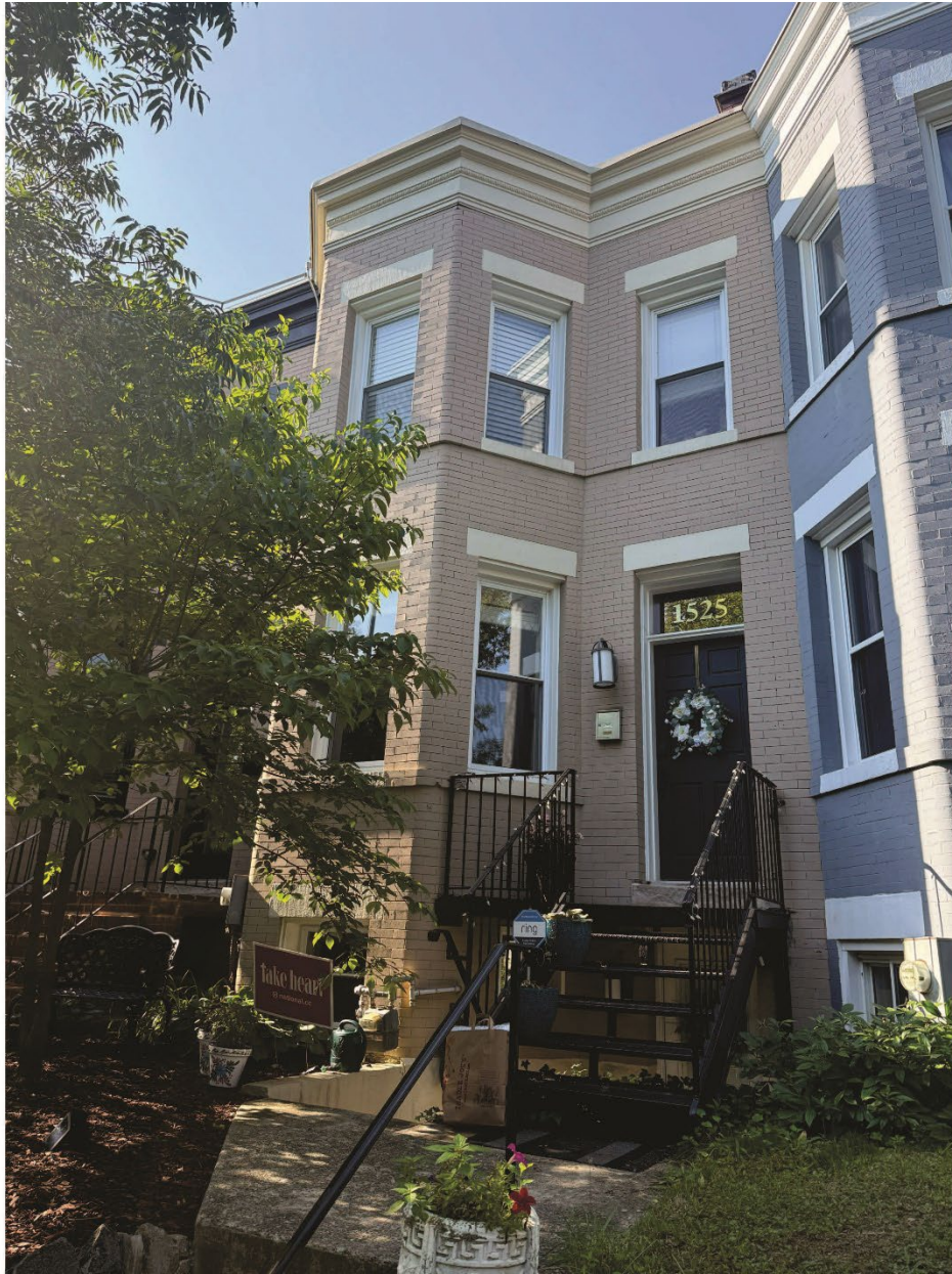
View of Property Frontage 1525 A Street NE
