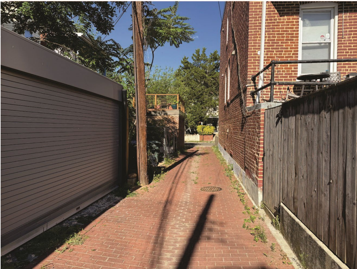
Eastward down the alley from the Property
