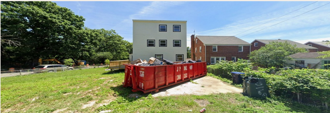
Rear yard, facing the alley
