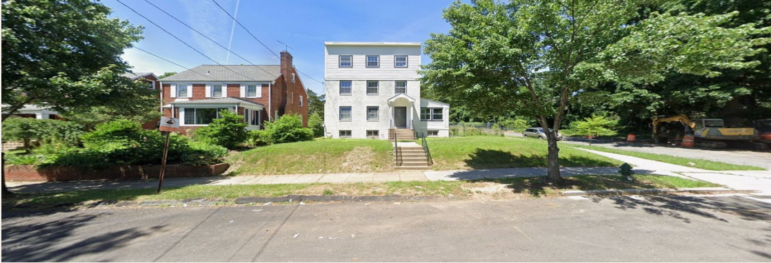
Front (east) elevation from 17th Street NE
