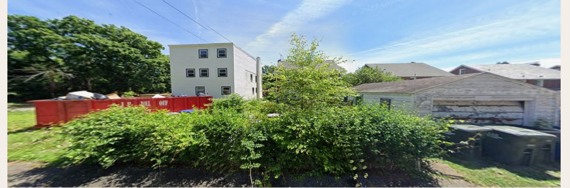
Side (north/rear) elevation, existing conditions
